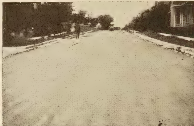
FIGURE 62.—SURFACE TREATED LIMEROCK ROAD SIX INCHES THICK IN FLORIDA
